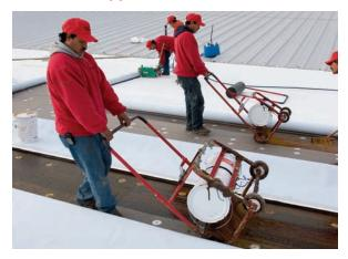
UltraPlyTPO XR can be fully adhered, using environmentally friendly XR Bonding Adhesive, applied with hot asphalt or mechanically attached.
